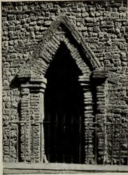
107. HOLY TRINITY, COLCHESTER. SAXON DOORWAY
